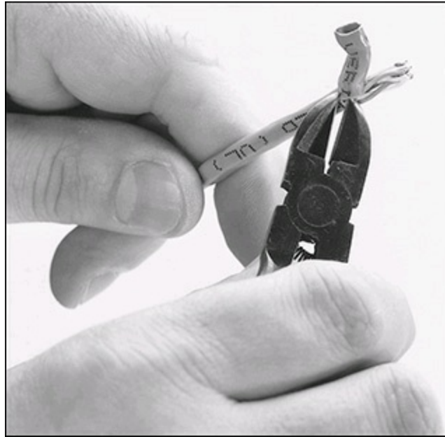
FIGURE 16.10 Carefully strip the cable jacket away to expose the four wire pairs.
