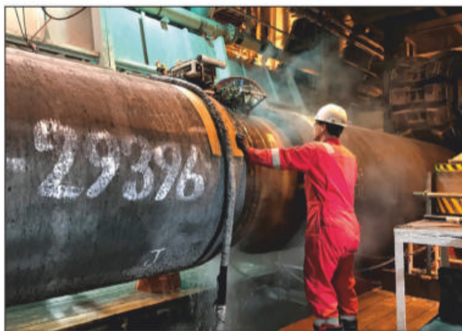
Preparing a pipe for the Nord Stream 2 project
