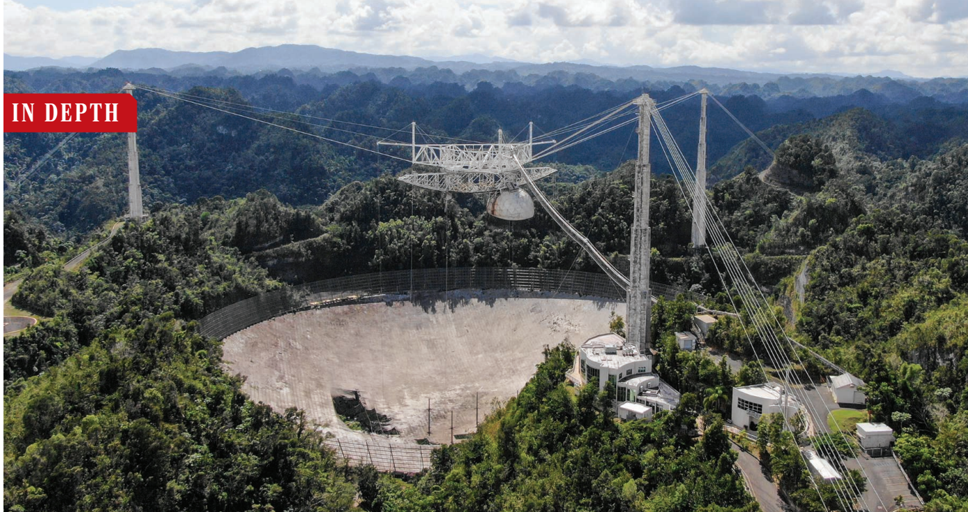
Broken suspension cables have torn through the Arecibo Observatory's dish panels and threaten to send the 900-ton instrument platform crashing down.
