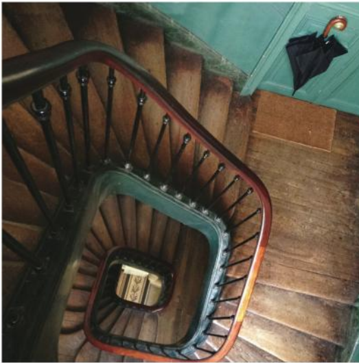
On the landing of an 18th-century Parisian staircase, an umbrella awaits the next walk in the rain. @TOMASVH
