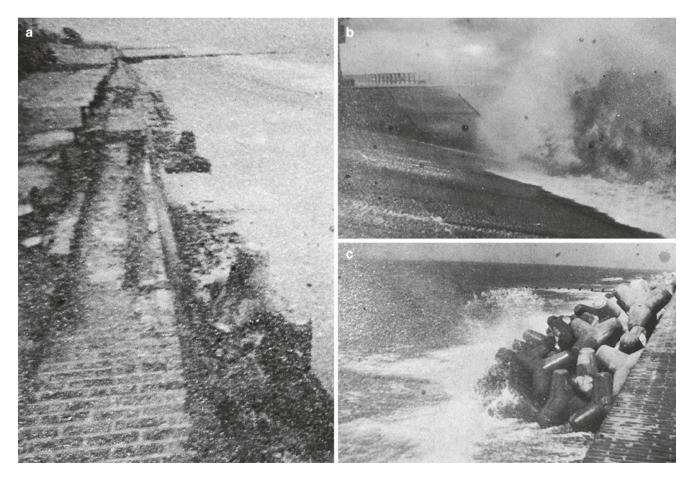
**Fig. 5.10** Defense against violent surf action in Westerland, Island of Sylt, German North Sea. (a) Damaged beach wall and displaced tetrapods; (b) gently sloping wall for breaking the power of storm waves;
